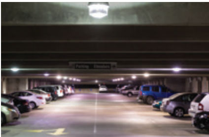
Before: Metal Halide Lighting
