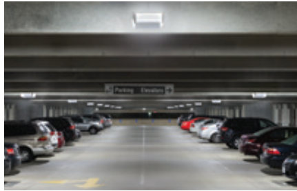
After: Cree WaveMax® Technology LED Lighting
