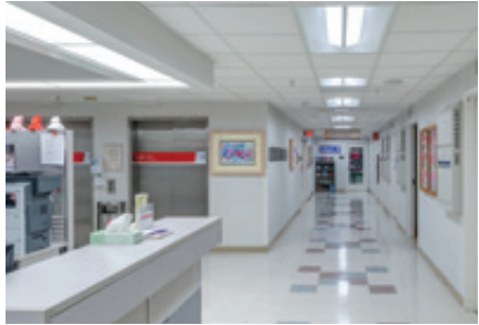
After: Cree TrueWhite® LED Lighting
